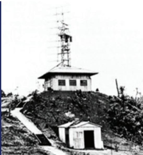
Early Radar Installation (SCR-271) in Panama
